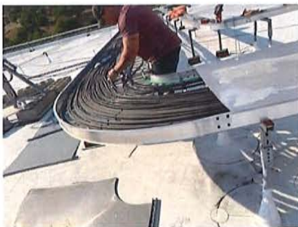
Installing Microwave cabling at the EOF site.
